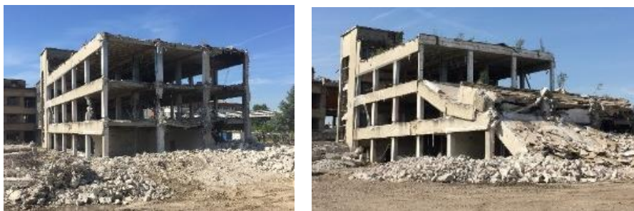
Before and after partial collapse
